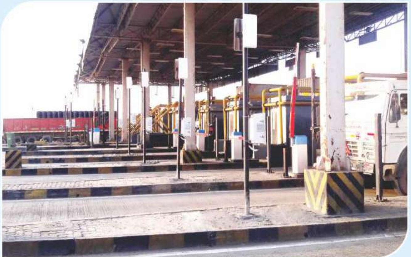
RFID readers installed at Toll Plazas under Logistics Data Service Project
