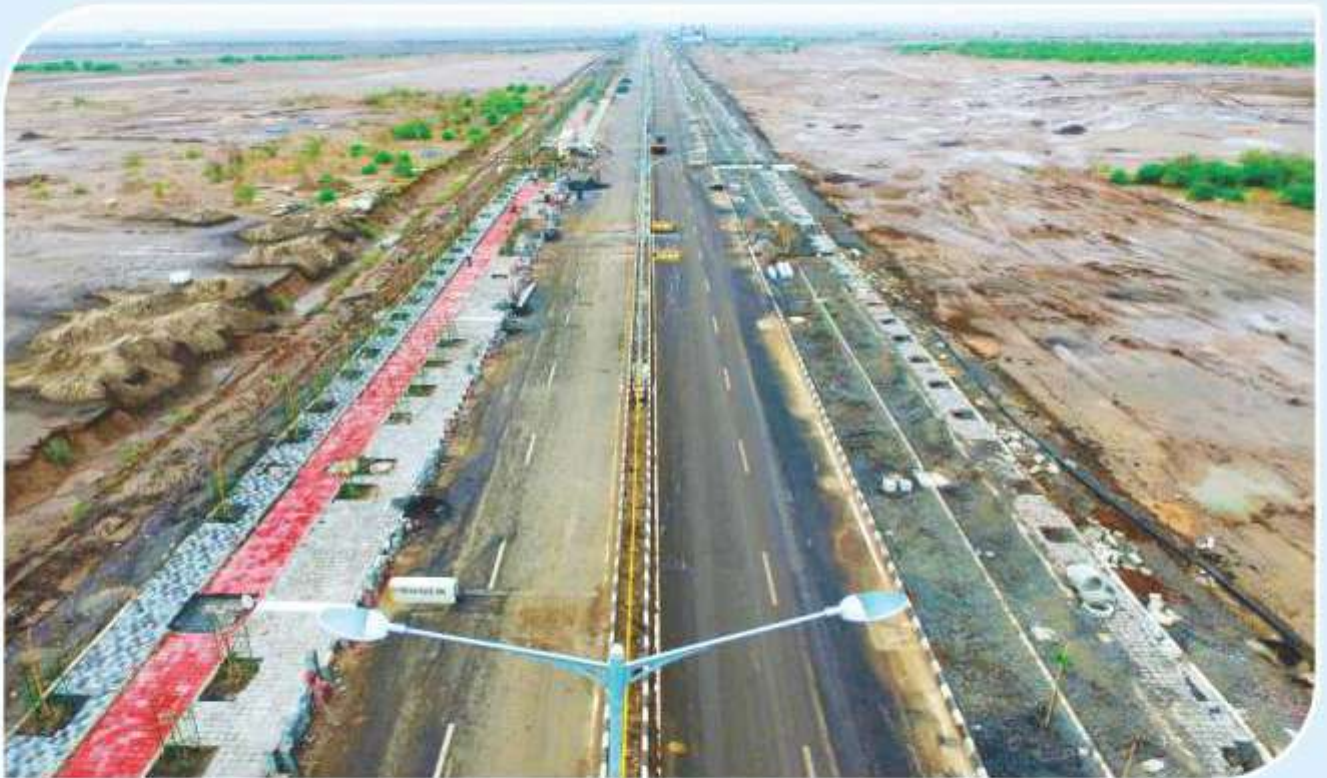
Construction of Roads and Services at Dholera, Gujrat
