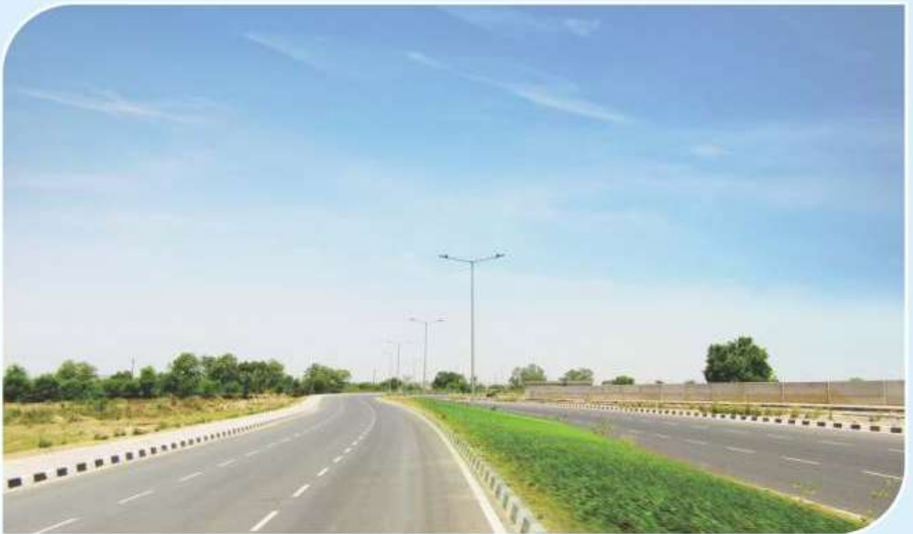
Road and Services at Integrated Industrial Township, at Greater Noida, UP
