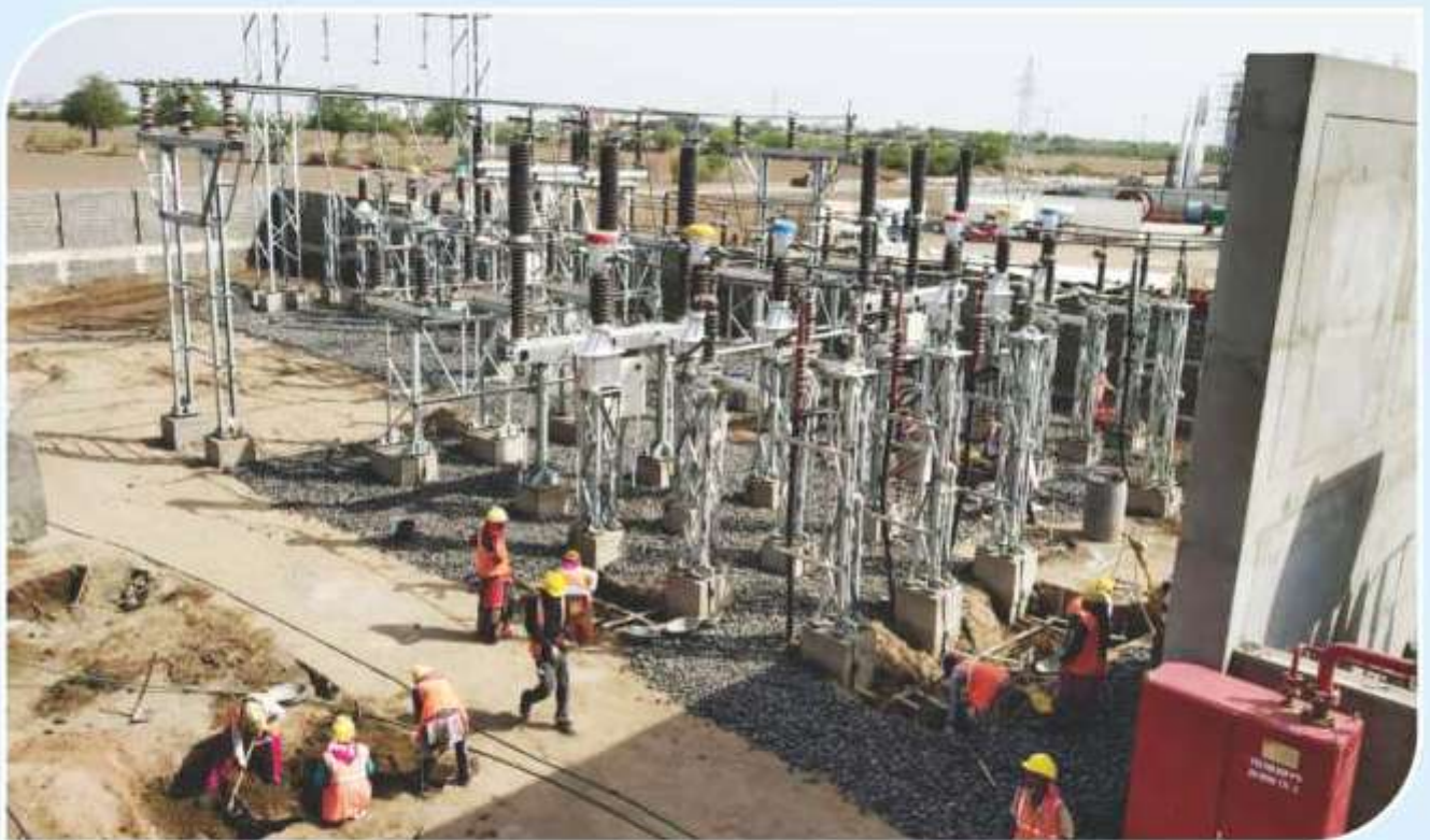
Construction of Sub-station by Torrent Power at Dholera, Gujarat
