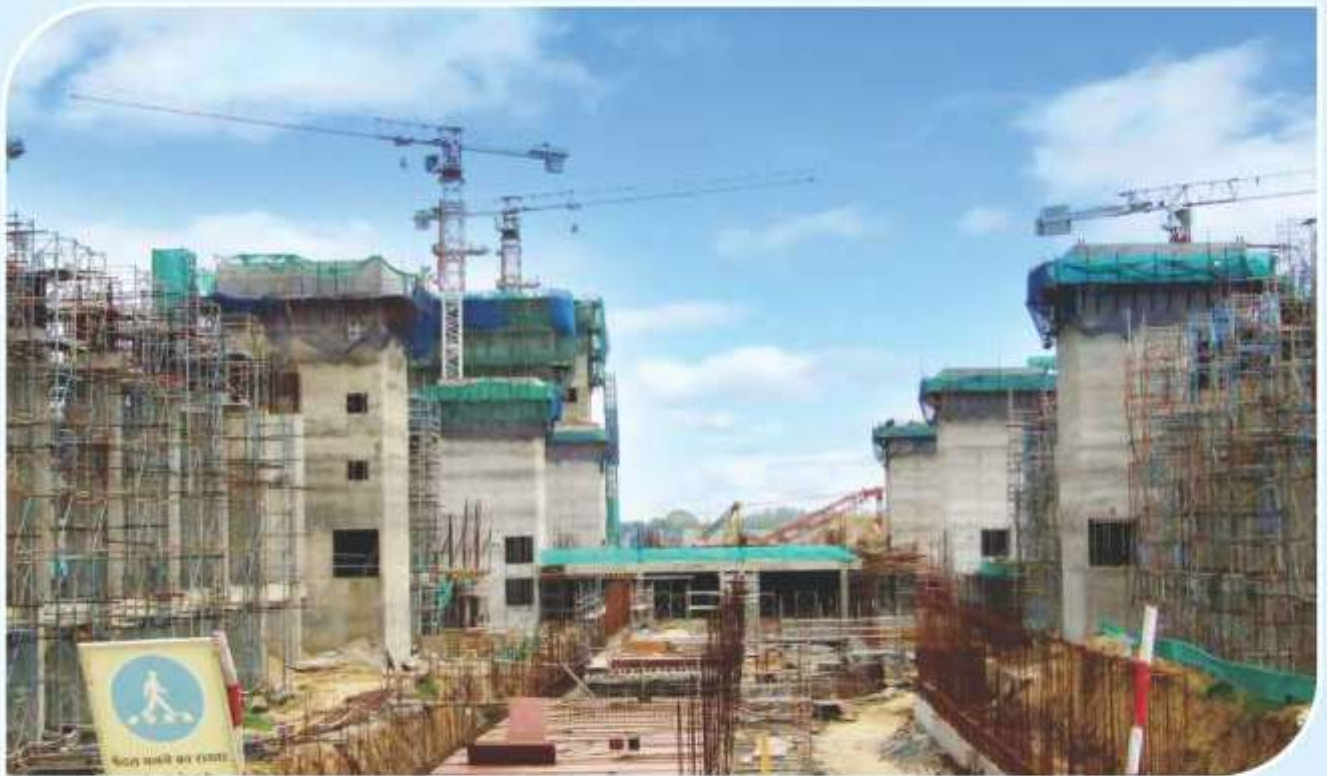
Construction activities in full swing at India International Exhibition and Convention Centre at Dwarka, New Delhi
