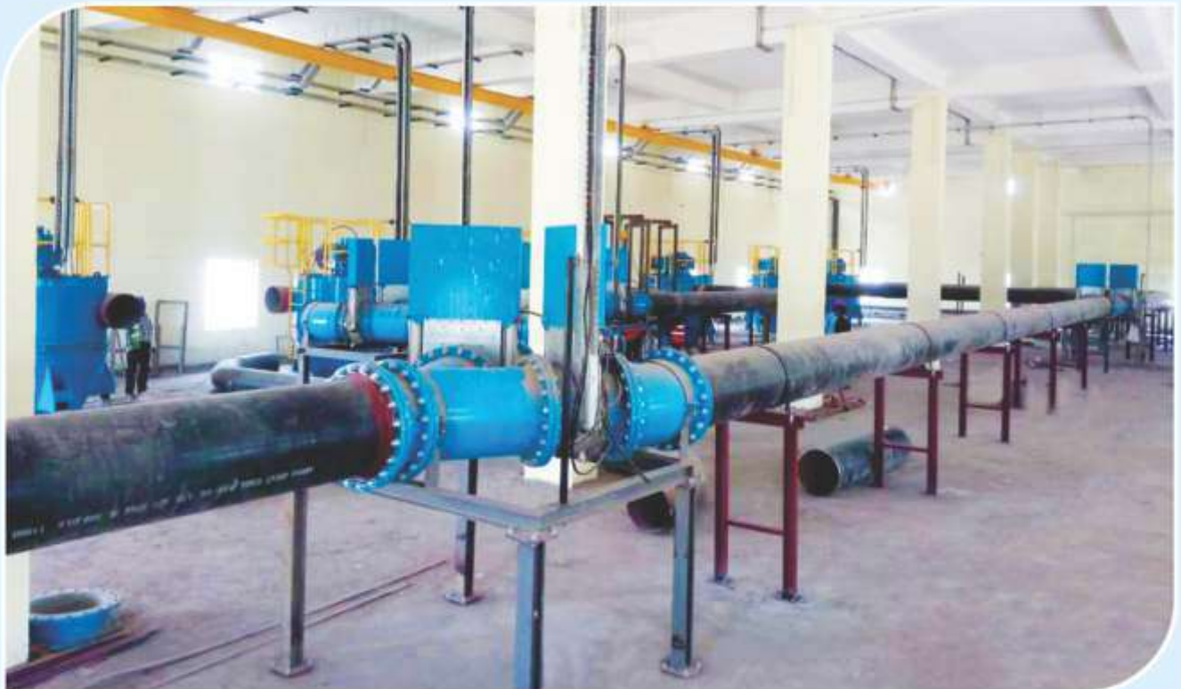
Automated Waste Collection System (AWCS) getting installed at Integrated Industrial Township at Greater Noida, U.P.
