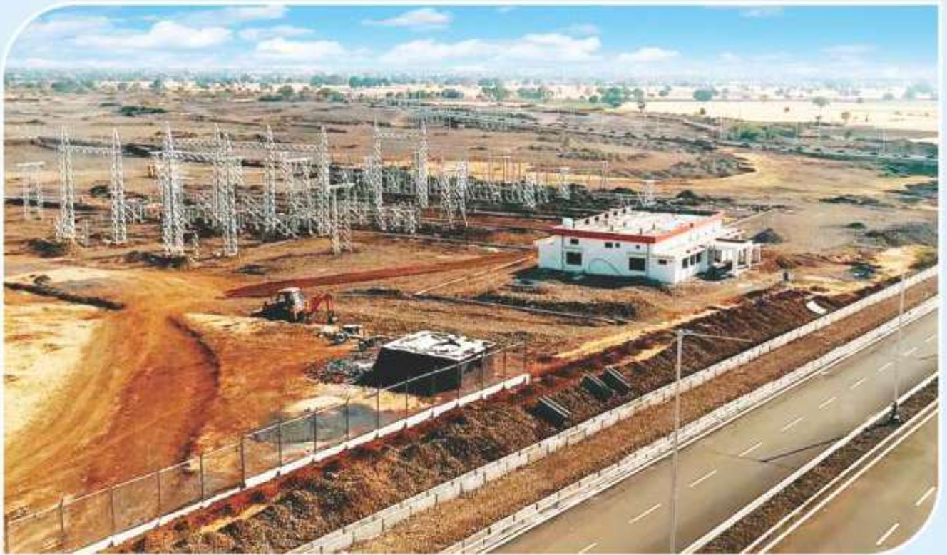
Construction activities in full swing at Integrated Industrial Township "Vikram Udyogpuri" near Ujjain, MP
