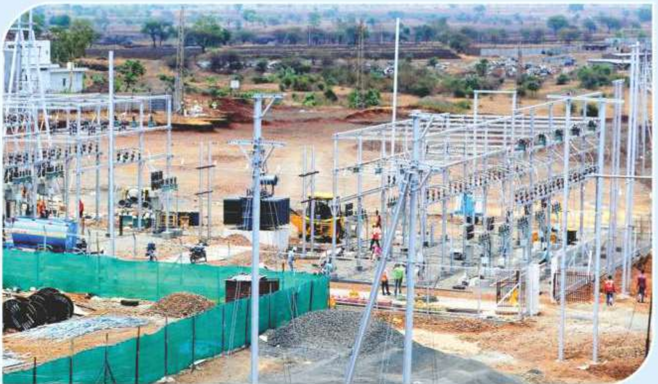
Construction of Sewage Treatment Plant and Power Sub-Station at Integrated Industrial Township "Vikram Udyogpuri" near Ujjain, MP
